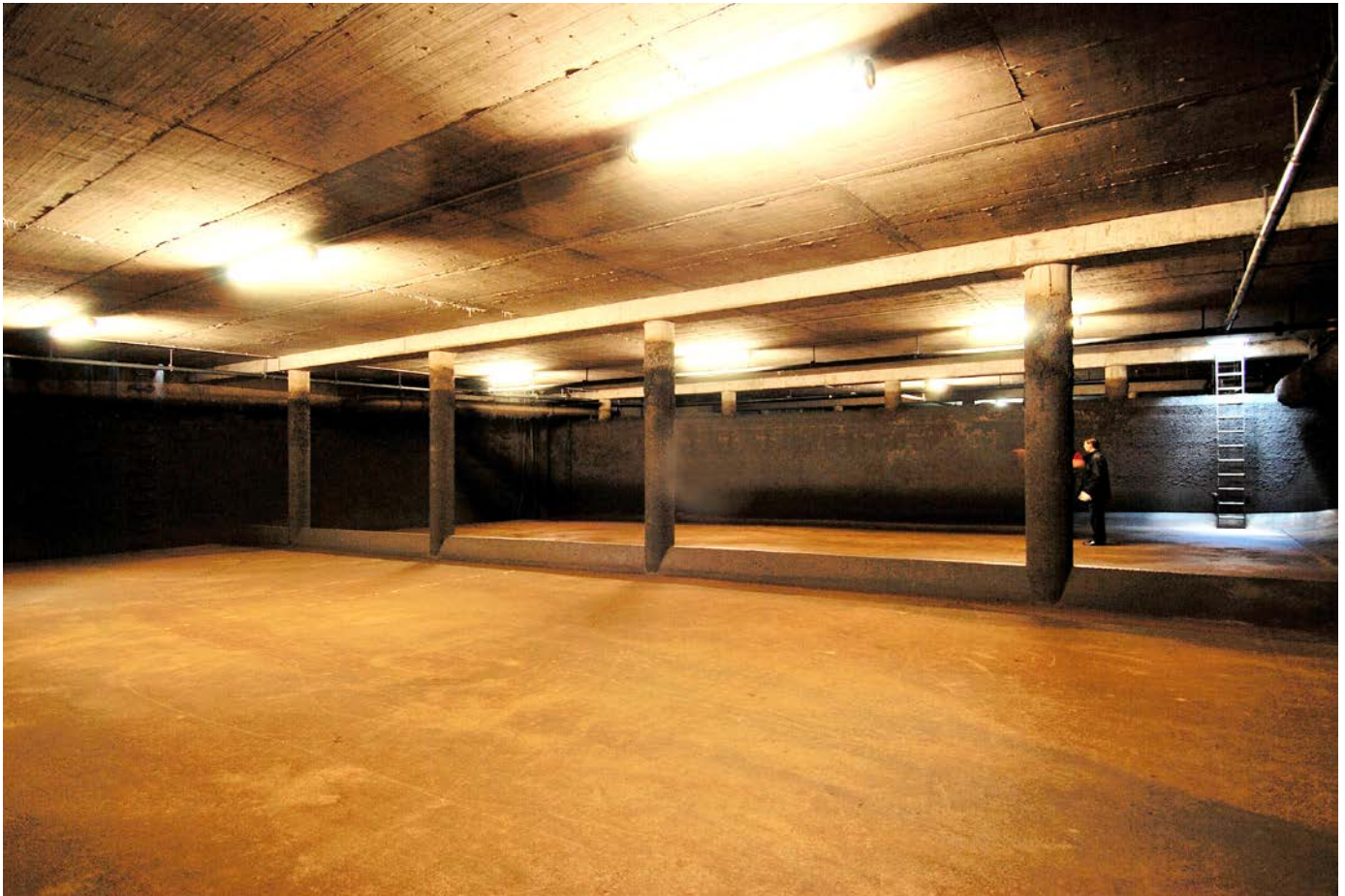
Rainwater recovery basin, Vlotho, Germany
