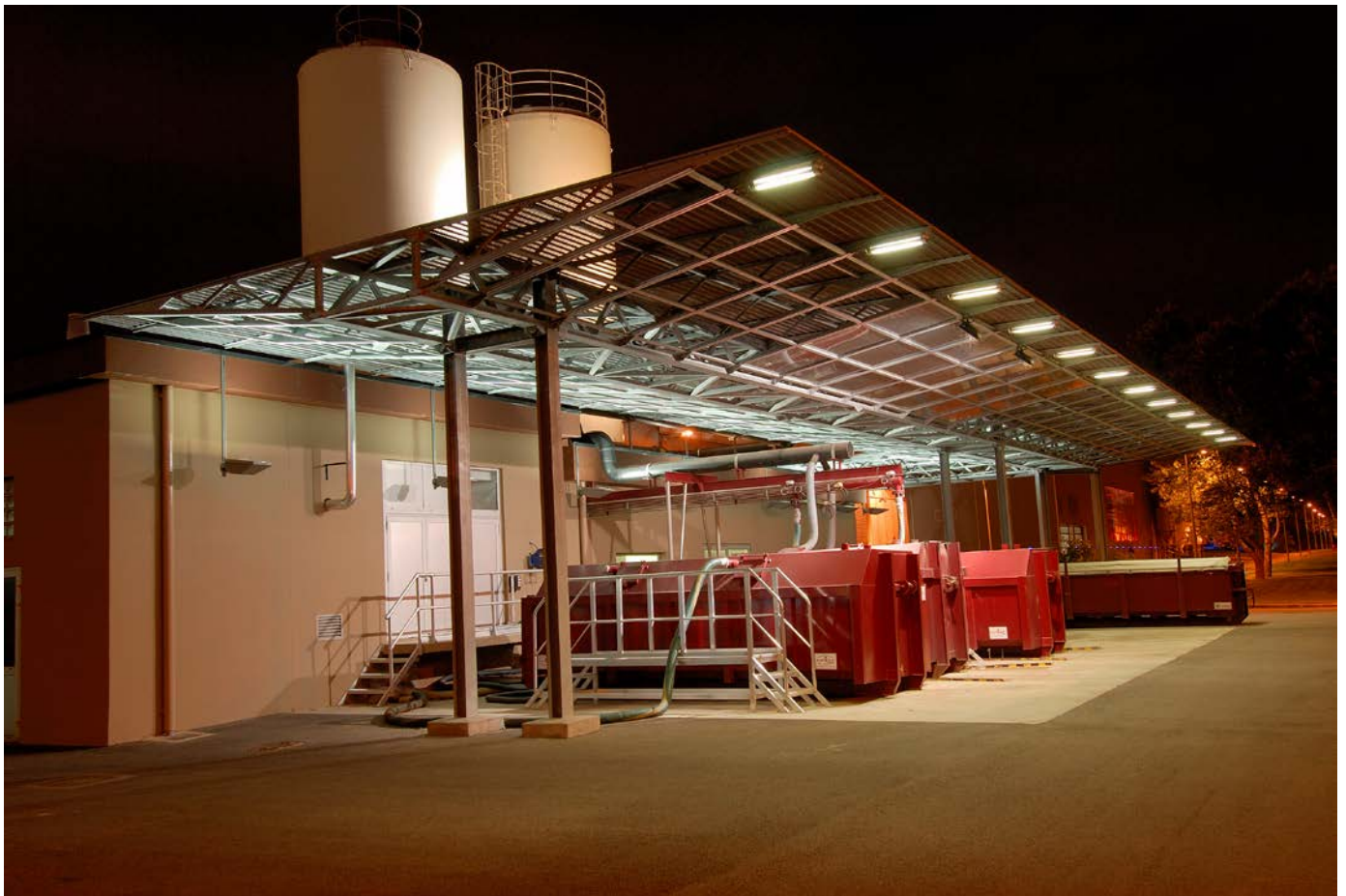
Wastewater treatment plant, Ginestous, France
